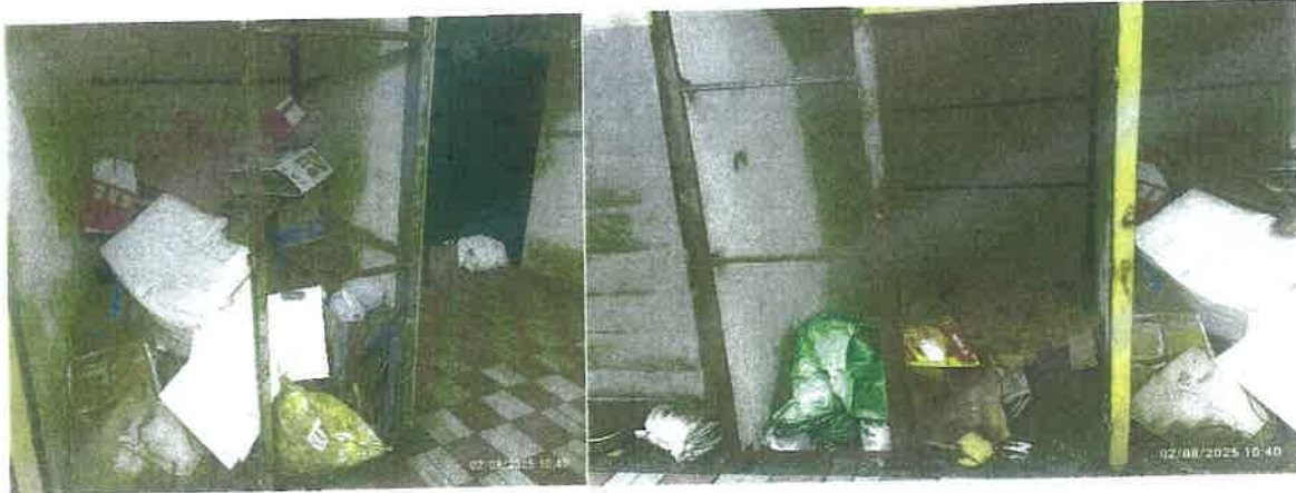
Staff Kitchen store/maintenance store/Garbage areas
