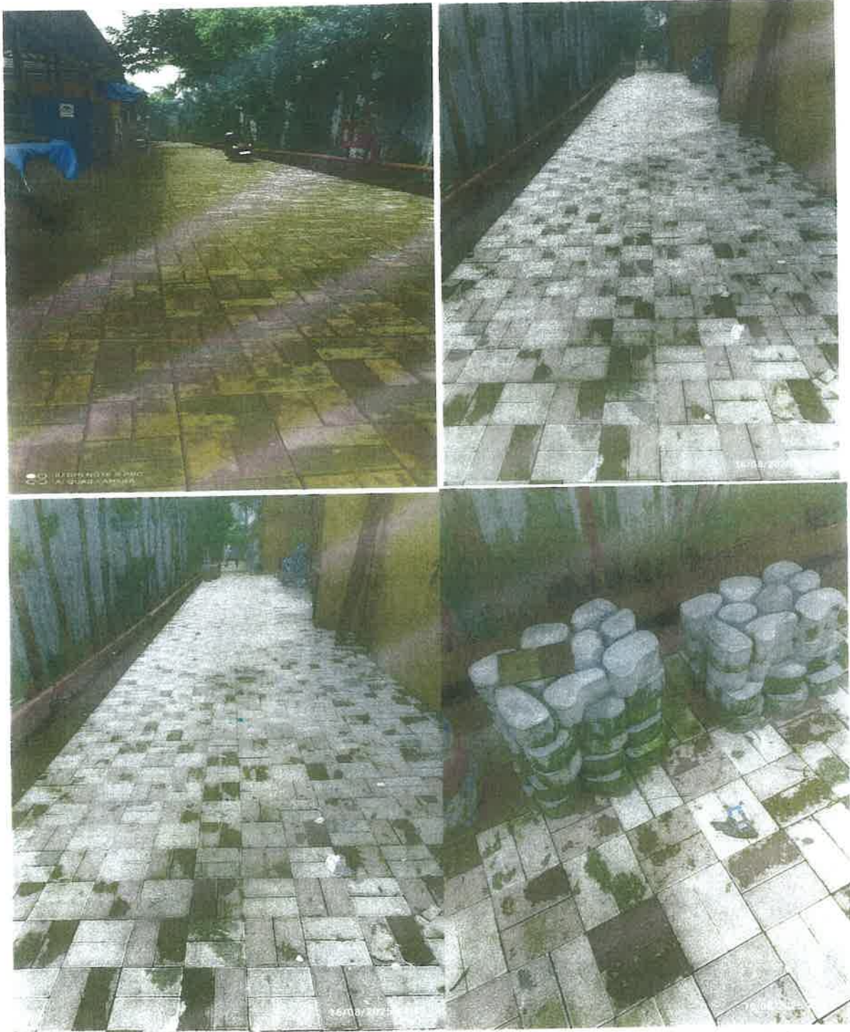
Pavers on the Service road to kitchen
